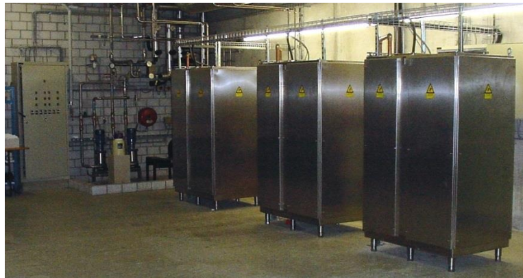
3 off x 30 kW 27.12MHz generators and their closed water cooling circuit
